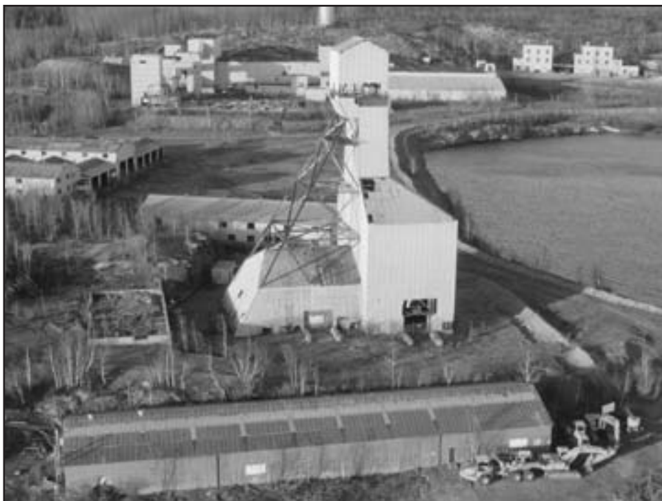
An aerial view of the buildings and structures left at the abandoned Gunnar Mine site. (Photo courtesy of the Saskatchewan Research Council)
